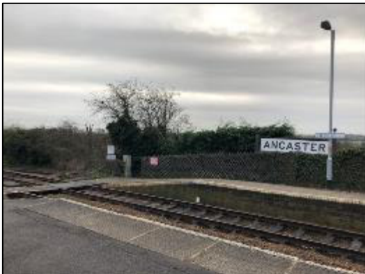
Photo: Station platforms with no tactiles and barrow crossing
