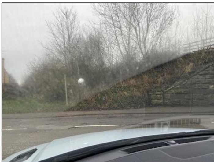
Photo (Eastbound): Station Approach egress onto Ermine Street, ineffective mirror opposite
